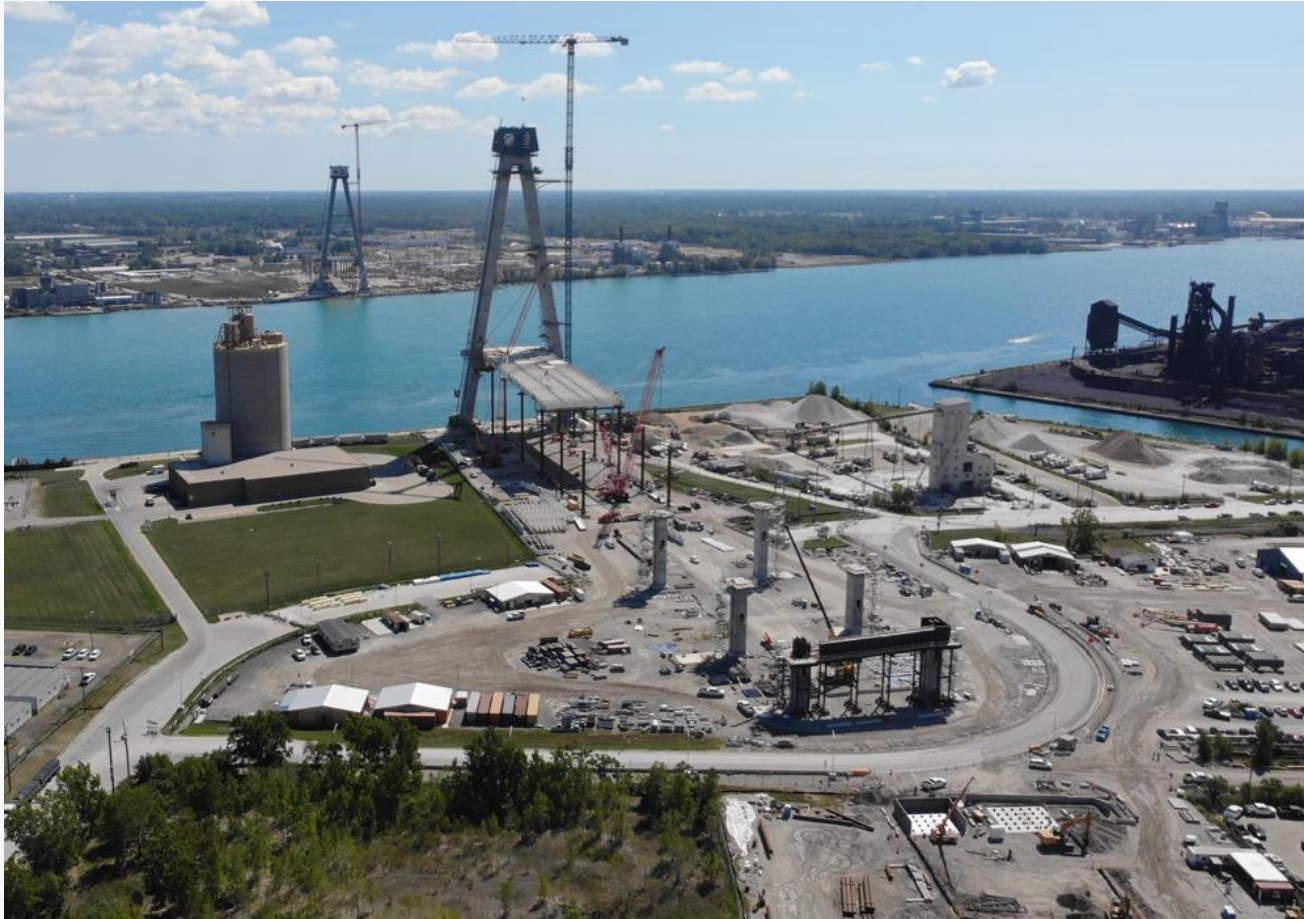
US bridge site back span and bridge towers
