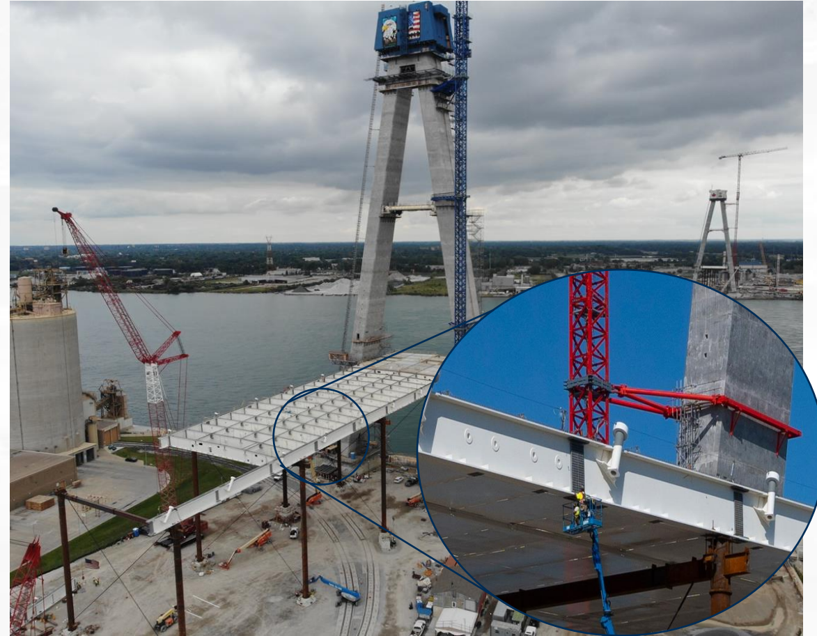
US bridge deck girder installation
