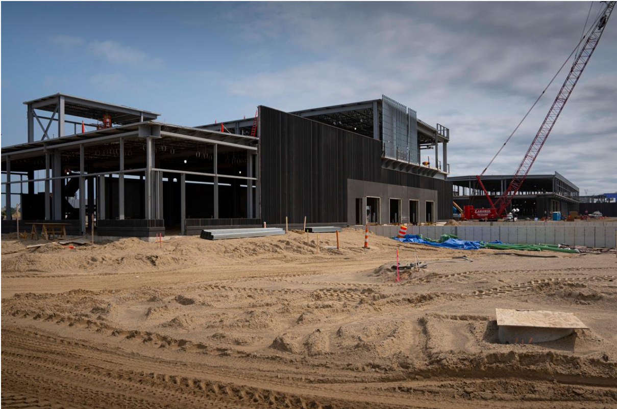
US POE building construction
