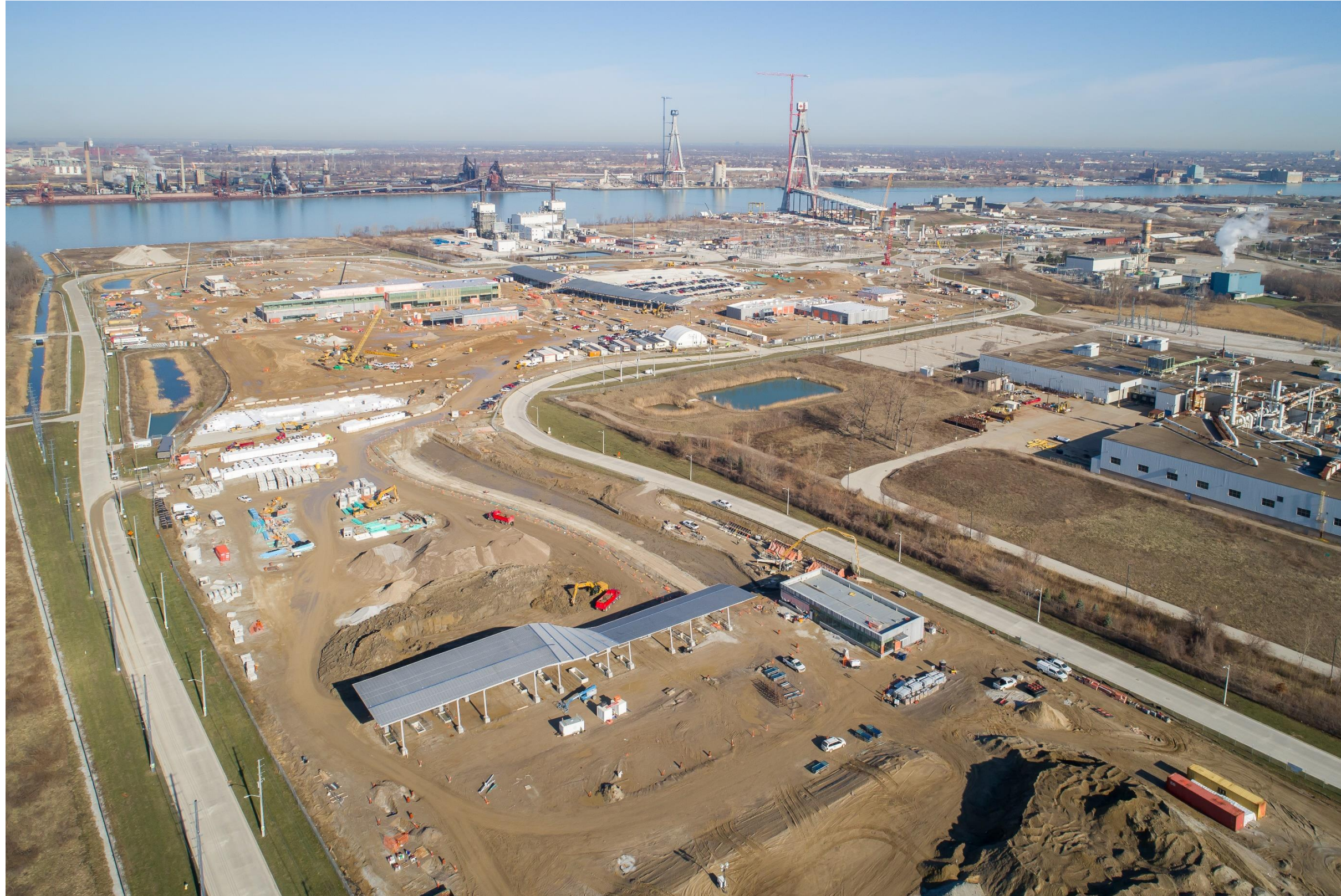
Canadian Port of Entry construction progress
