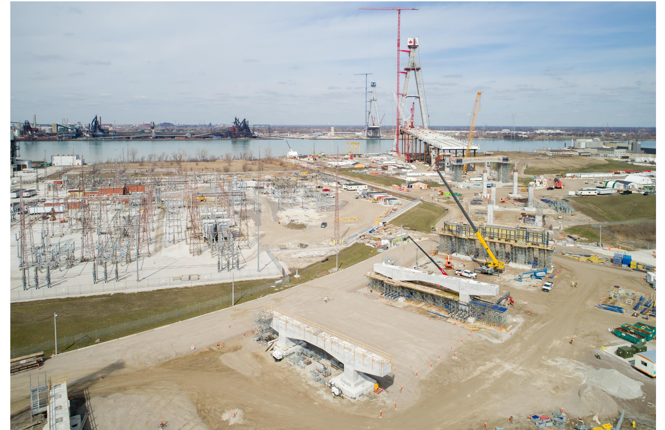
Canadian bridge site construction progress
