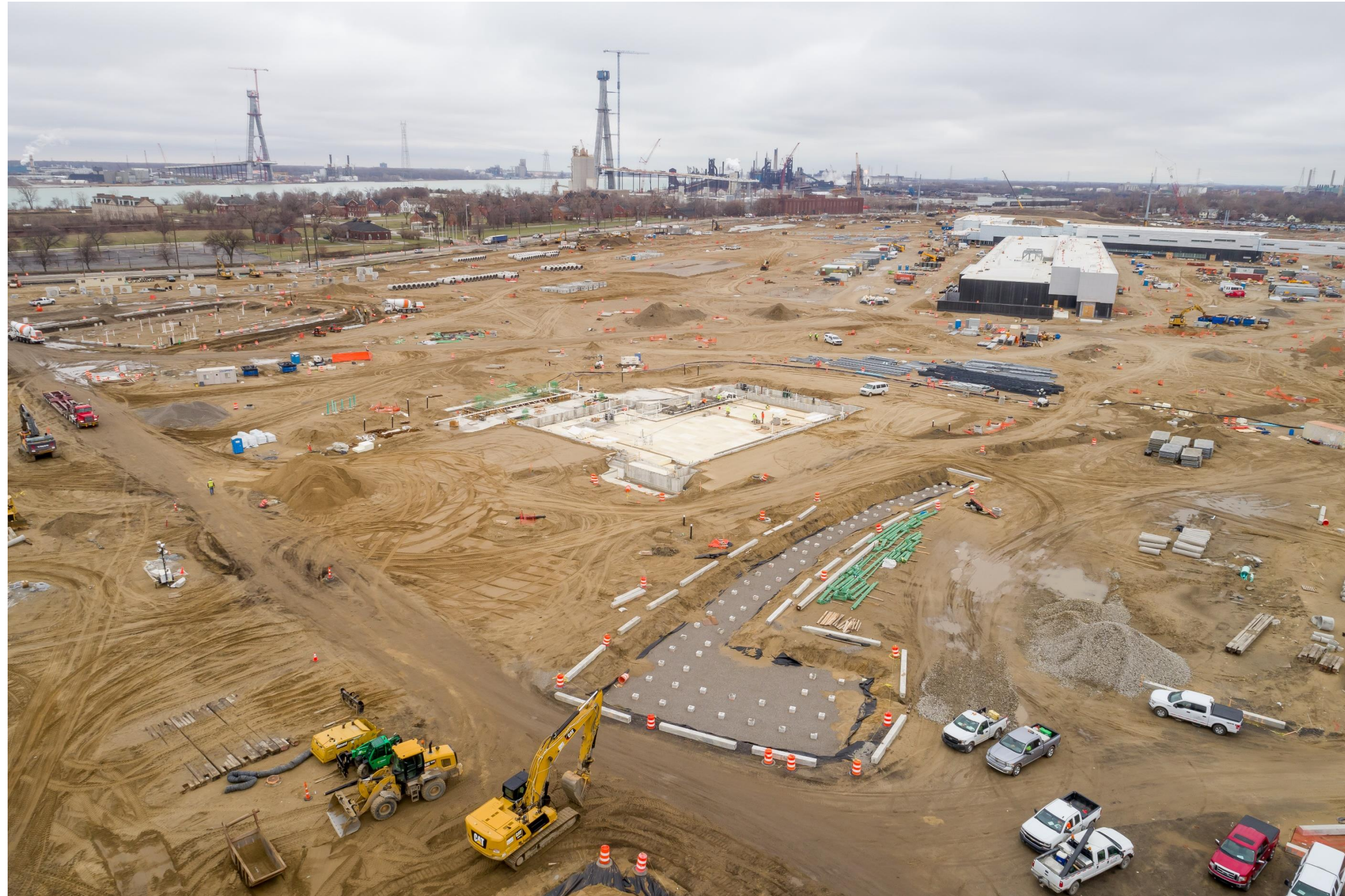
US Port of Entry construction progress
