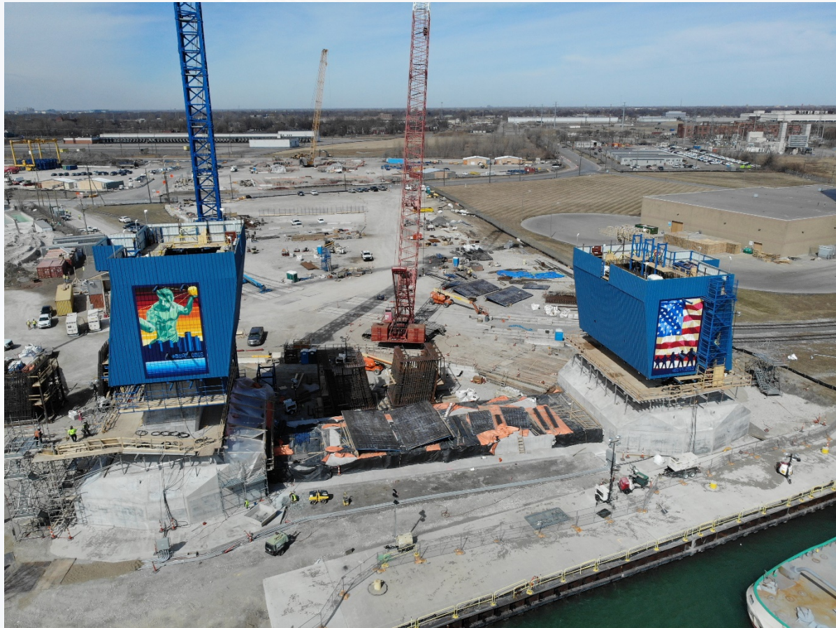
US bridge site tower work
