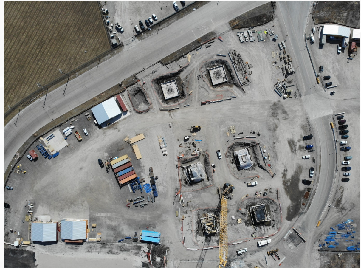
US bridge site side/back span work
