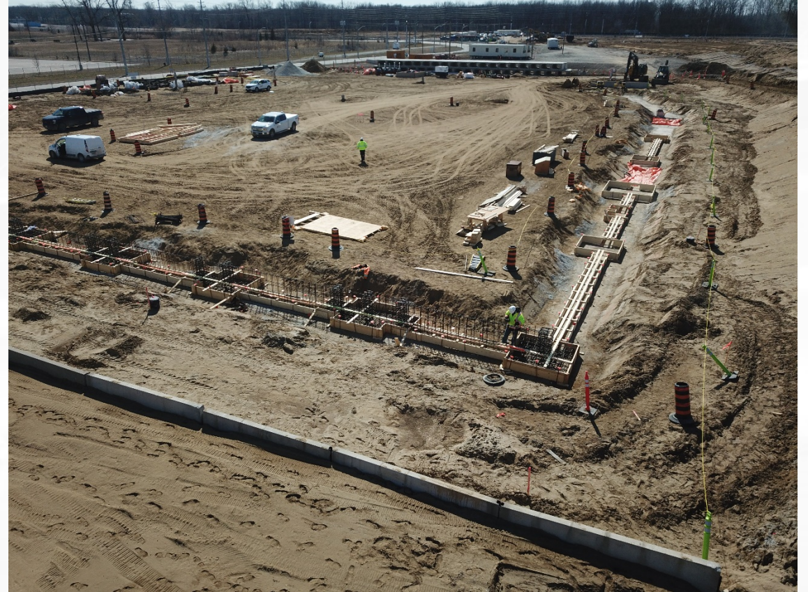
Canadian Port of Entry building foundations
