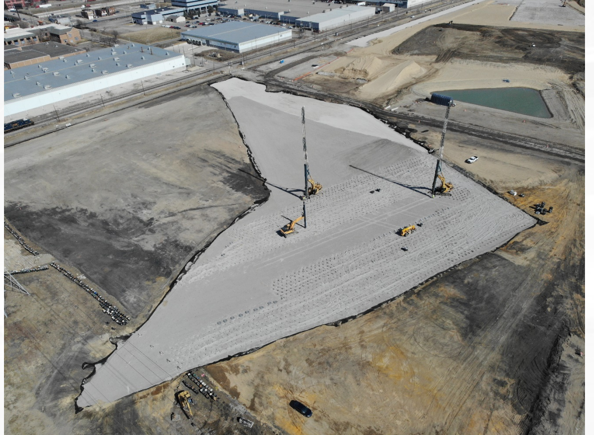
US Port of Entry wick drain installation
