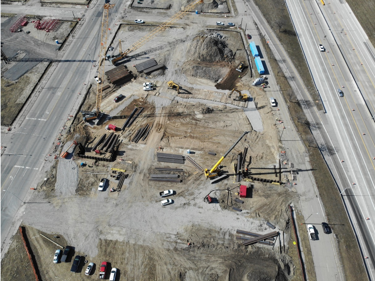
Michigan Interchange Cavalry siphon work
