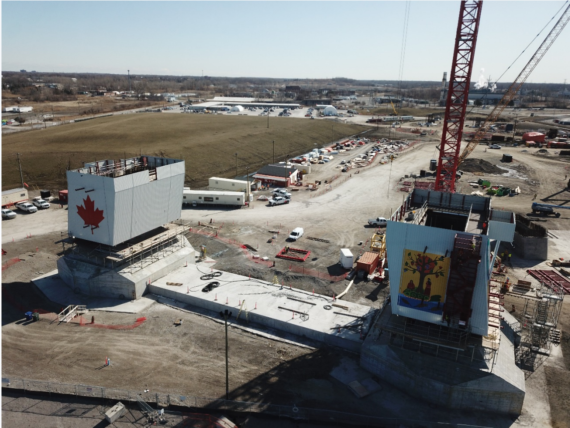
Canadian bridge site tower work
