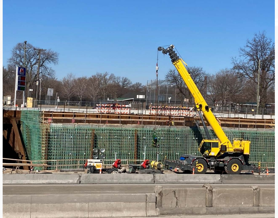
Michigan Interchange Clark bridge abutment work
