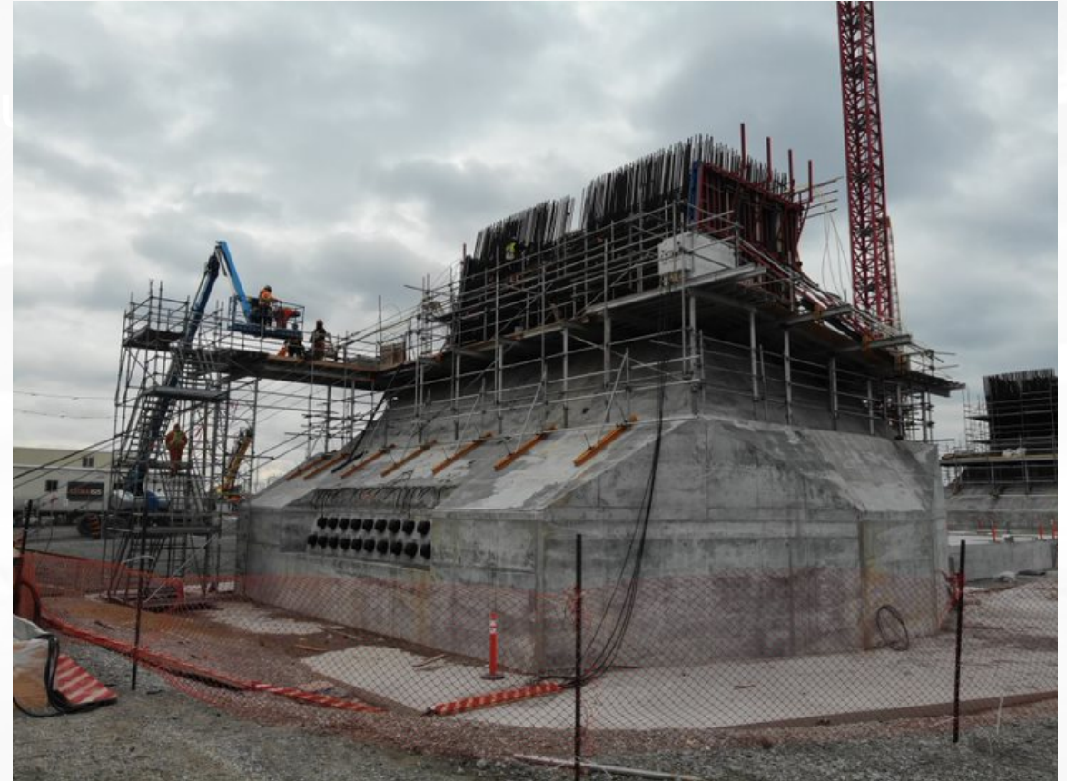
Canadian bridge site tower work
