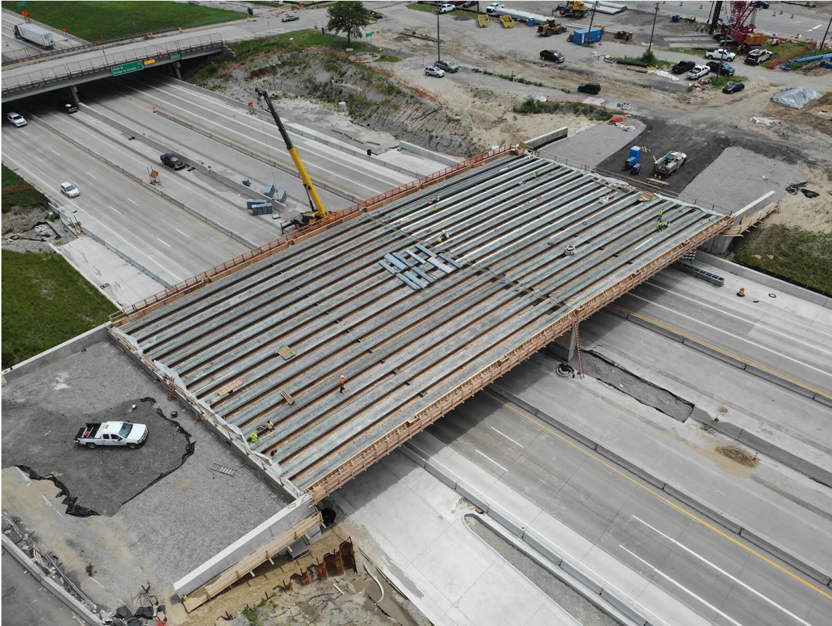
MI Interchange road bridge construction
