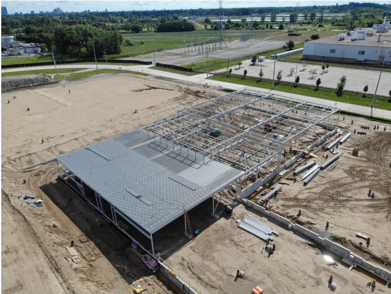
Canadian POE building construction
