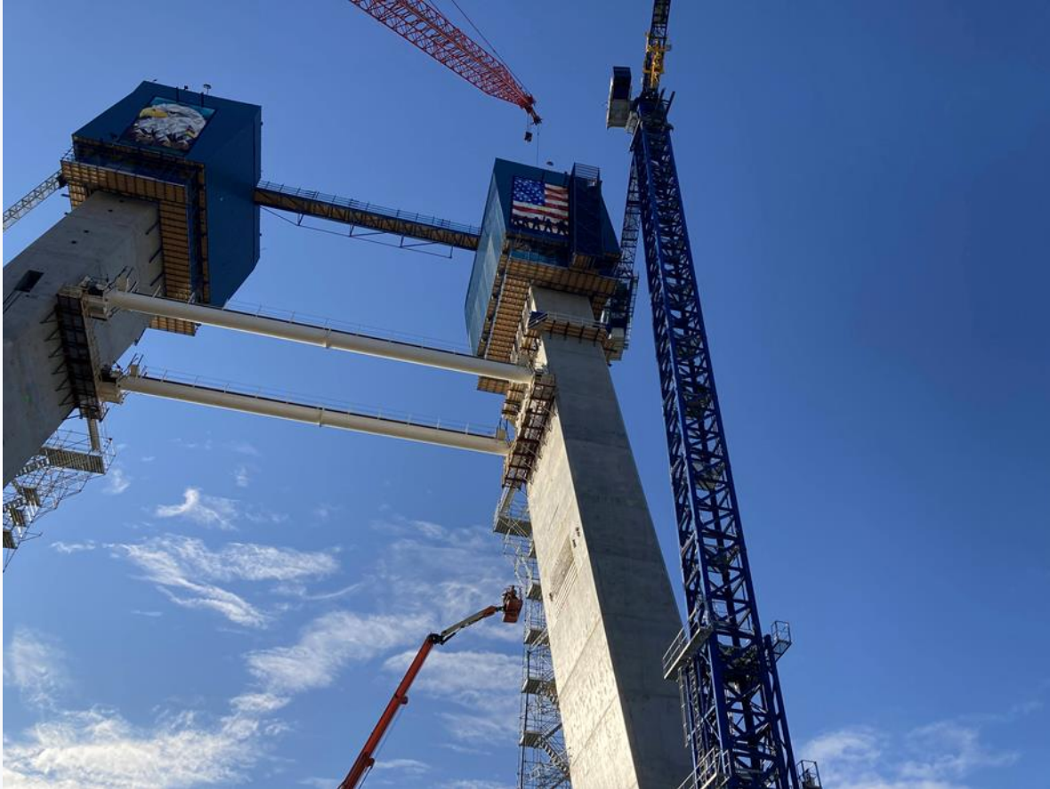
US bridge tower work
