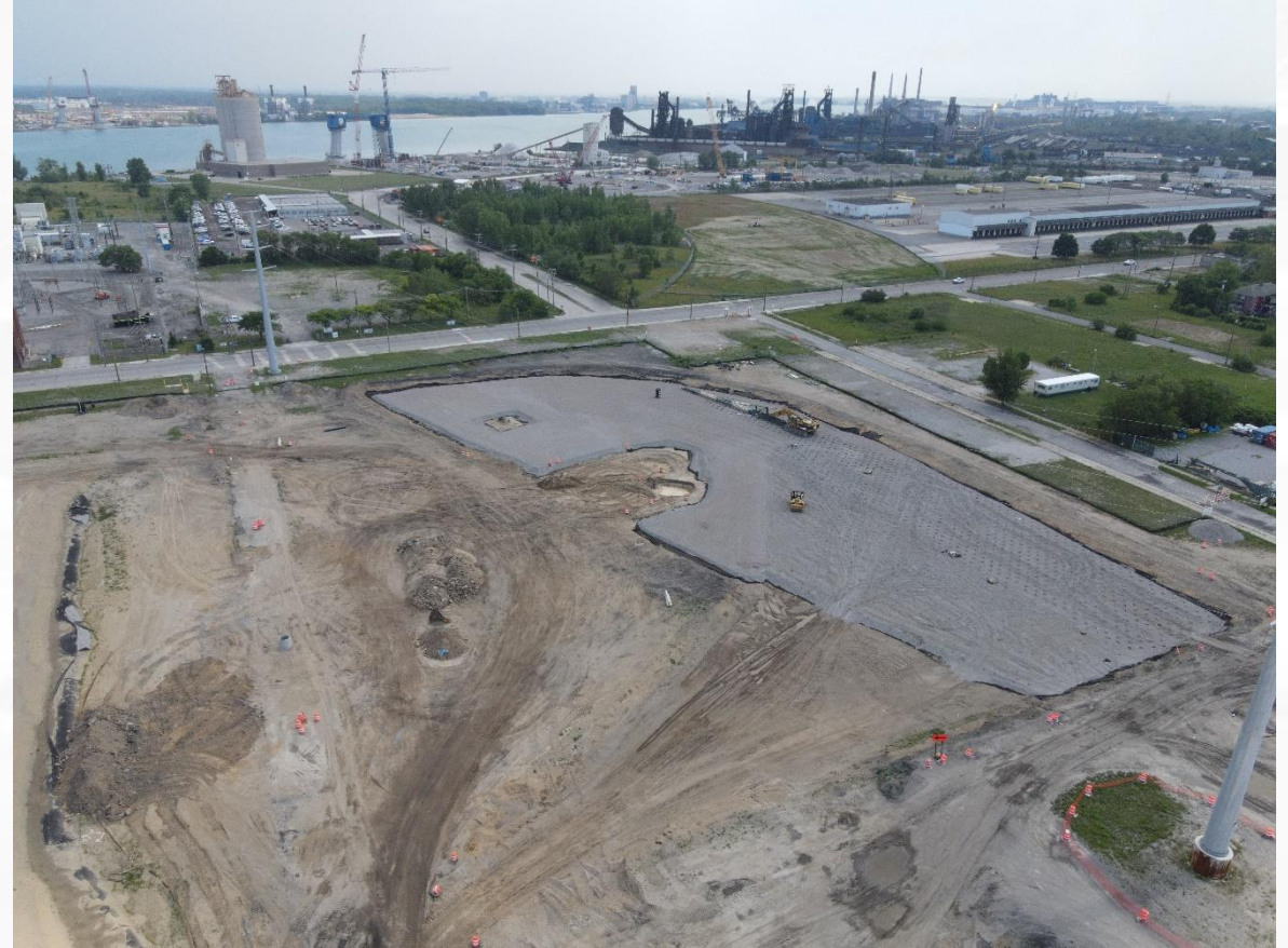
US POE wick drain installation
