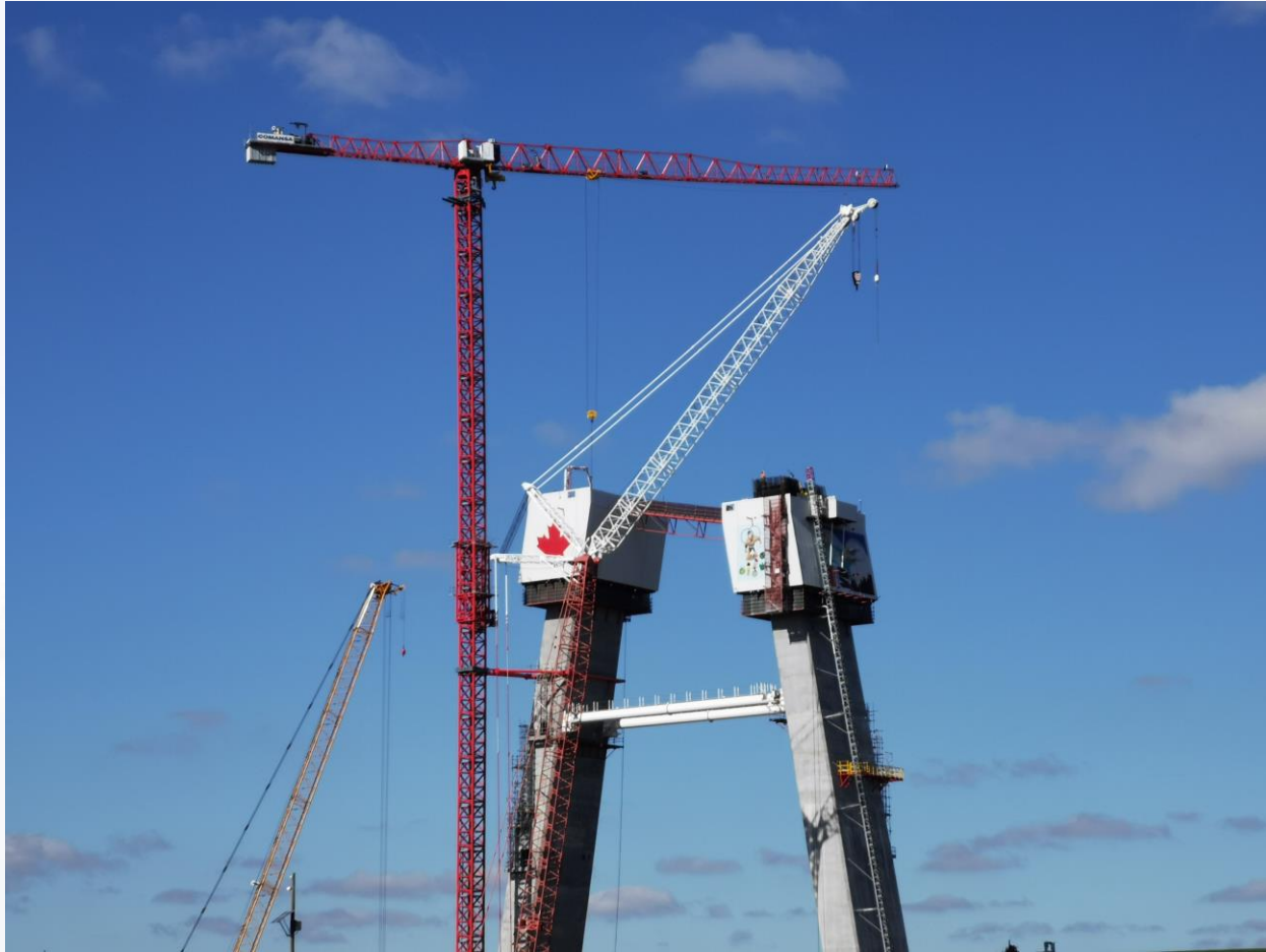
Canadian bridge tower work
