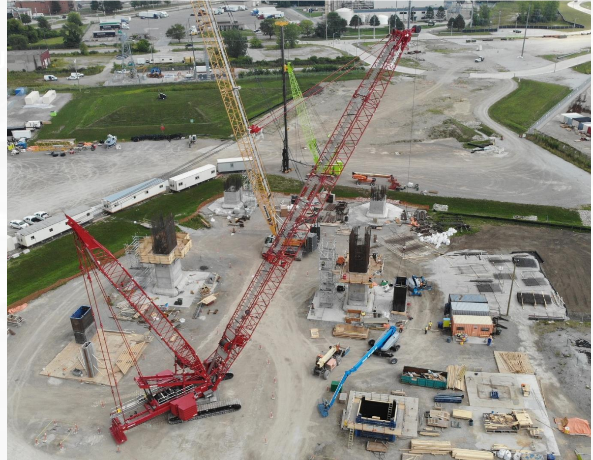
Canadian bridge back span tower work
