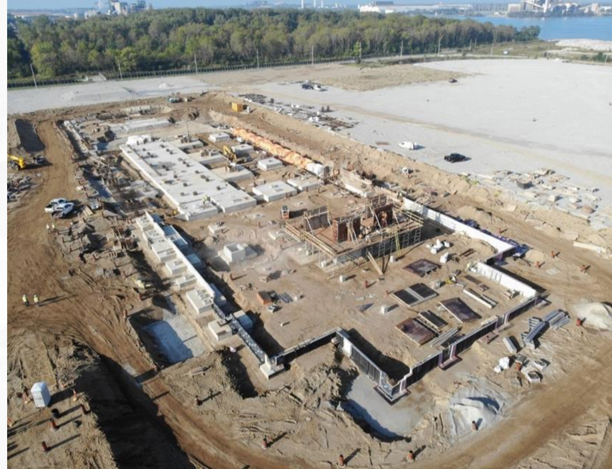
Canadian POE building construction
