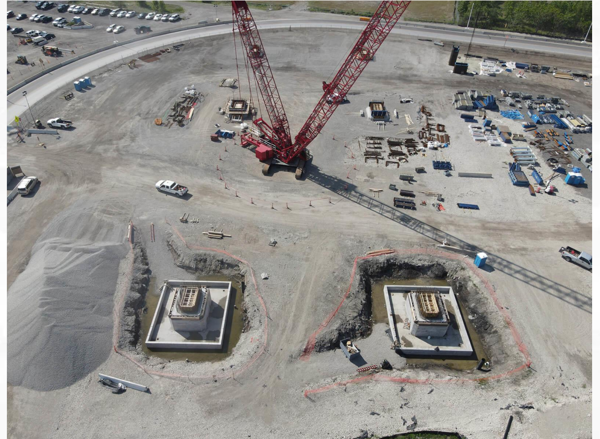
US bridge back span work
