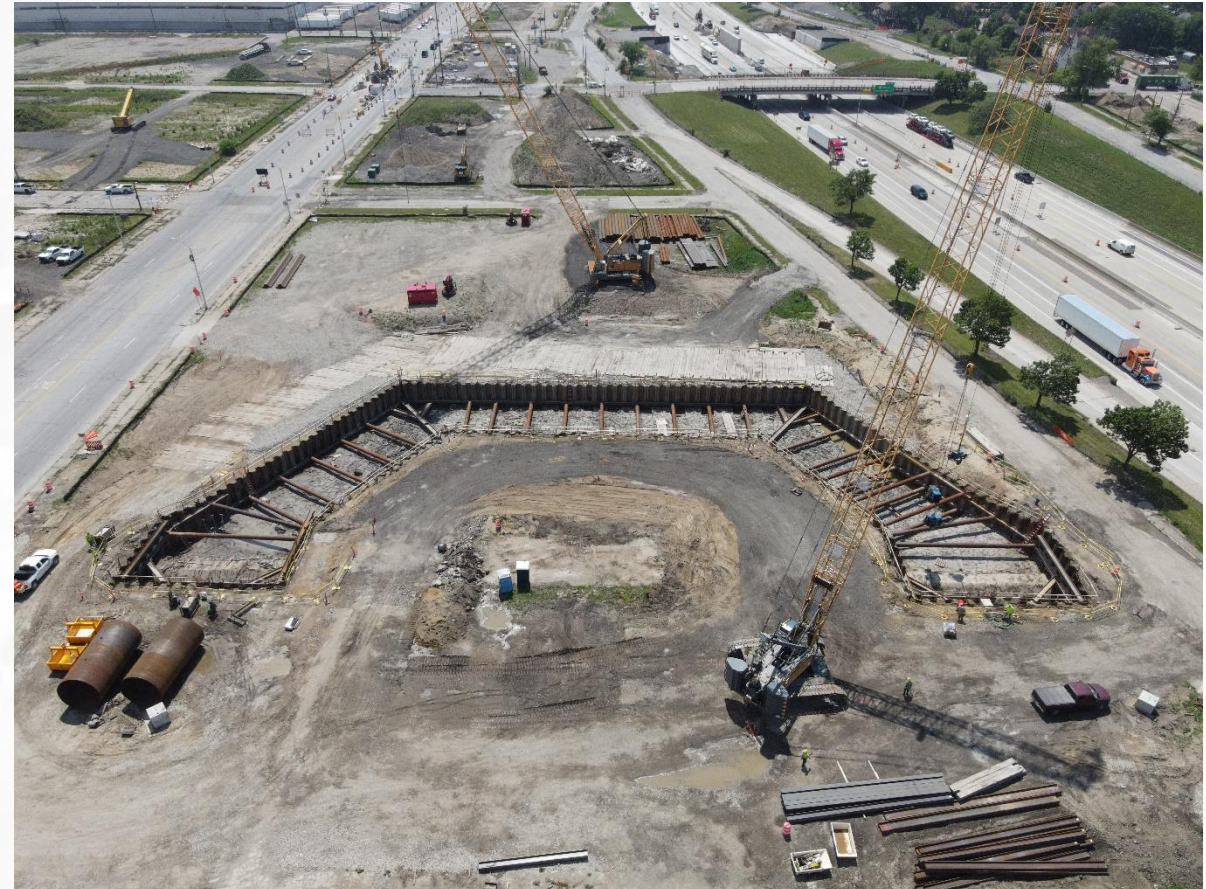
Cavalry siphon construction
