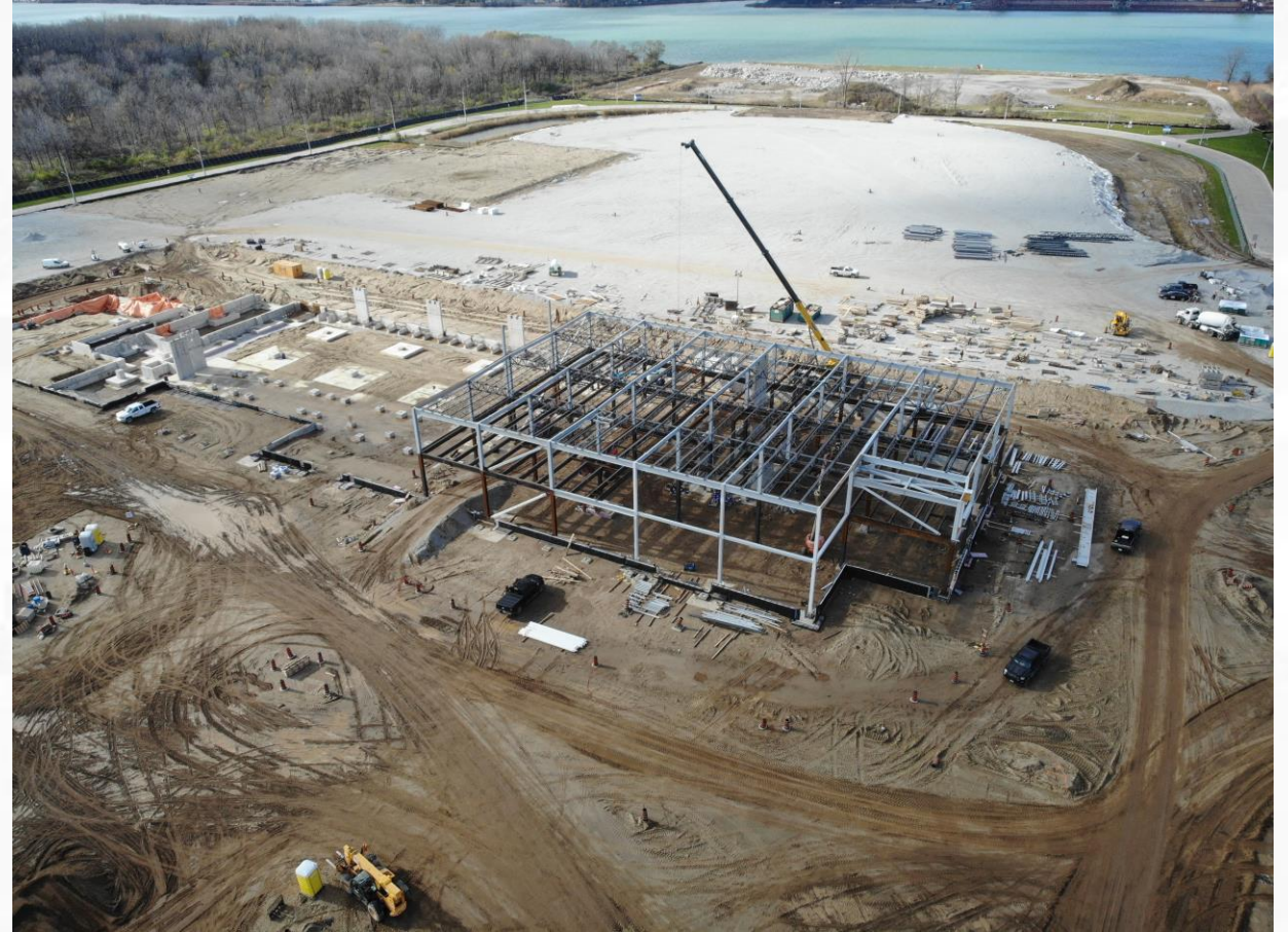
Canadian POE Main Building construction
