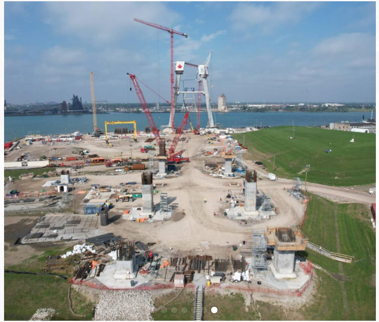
Canadian bridge back span tower work
