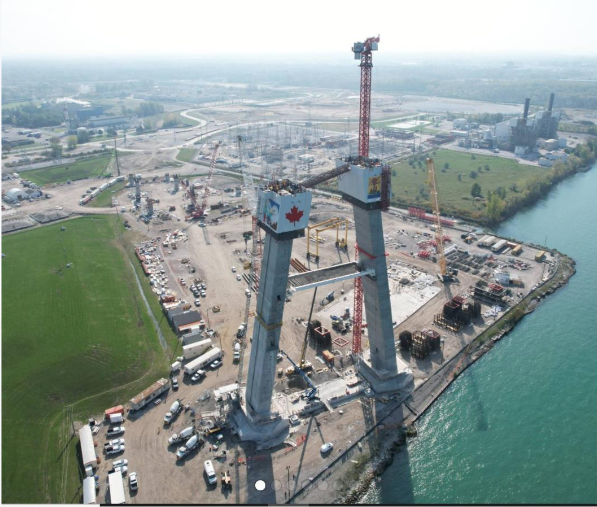
Canadian bridge tower work
