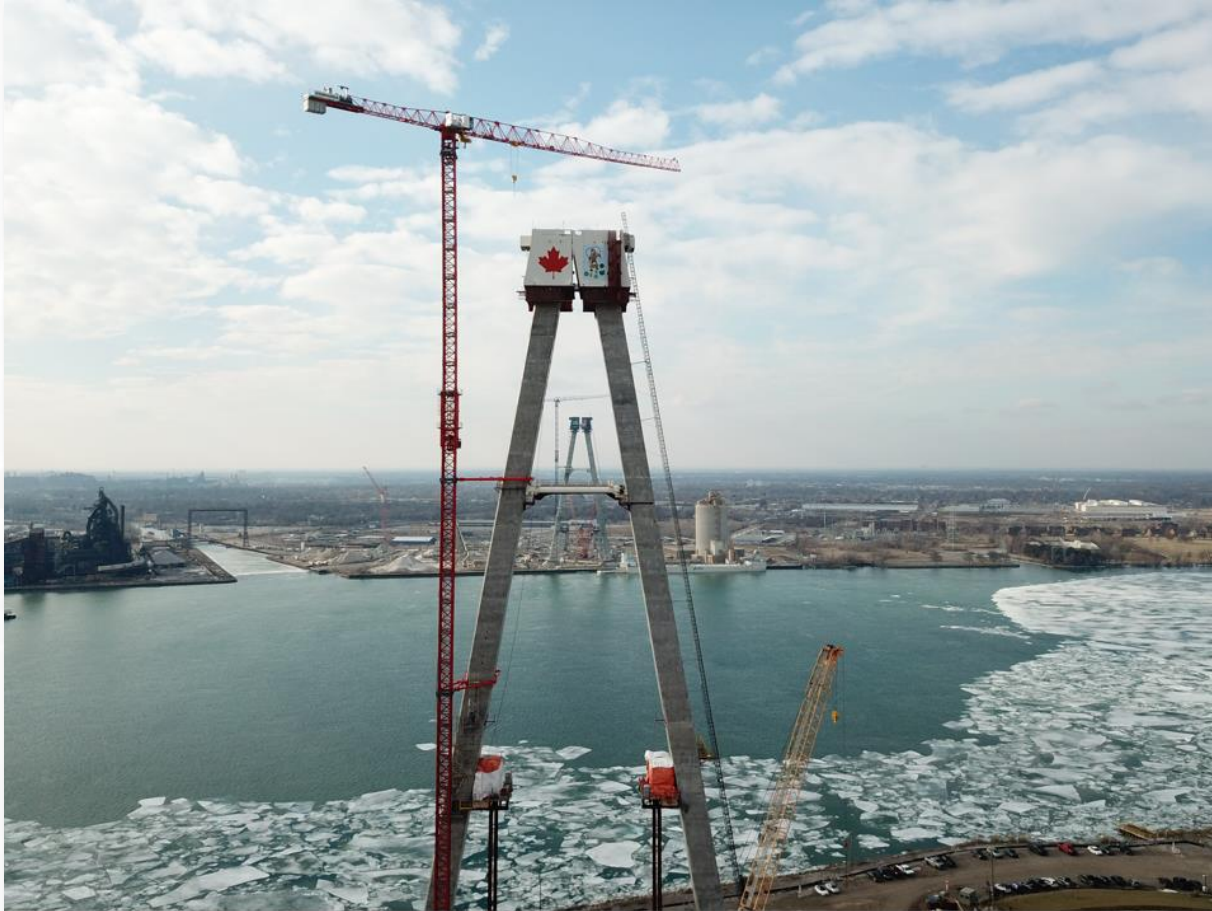
Canadian bridge tower work
