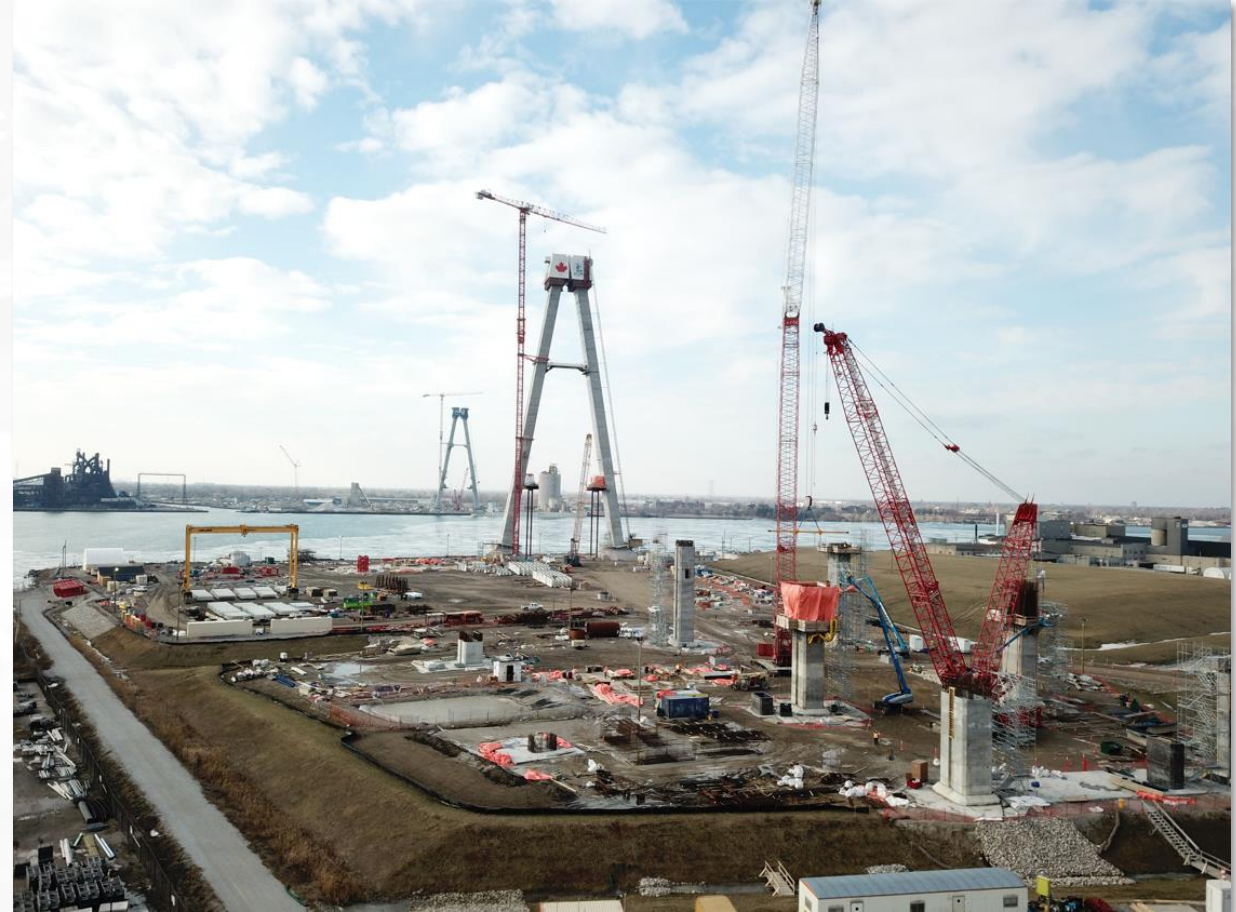
Canadian bridge back span work
