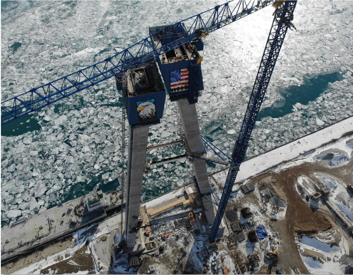
US bridge tower work
