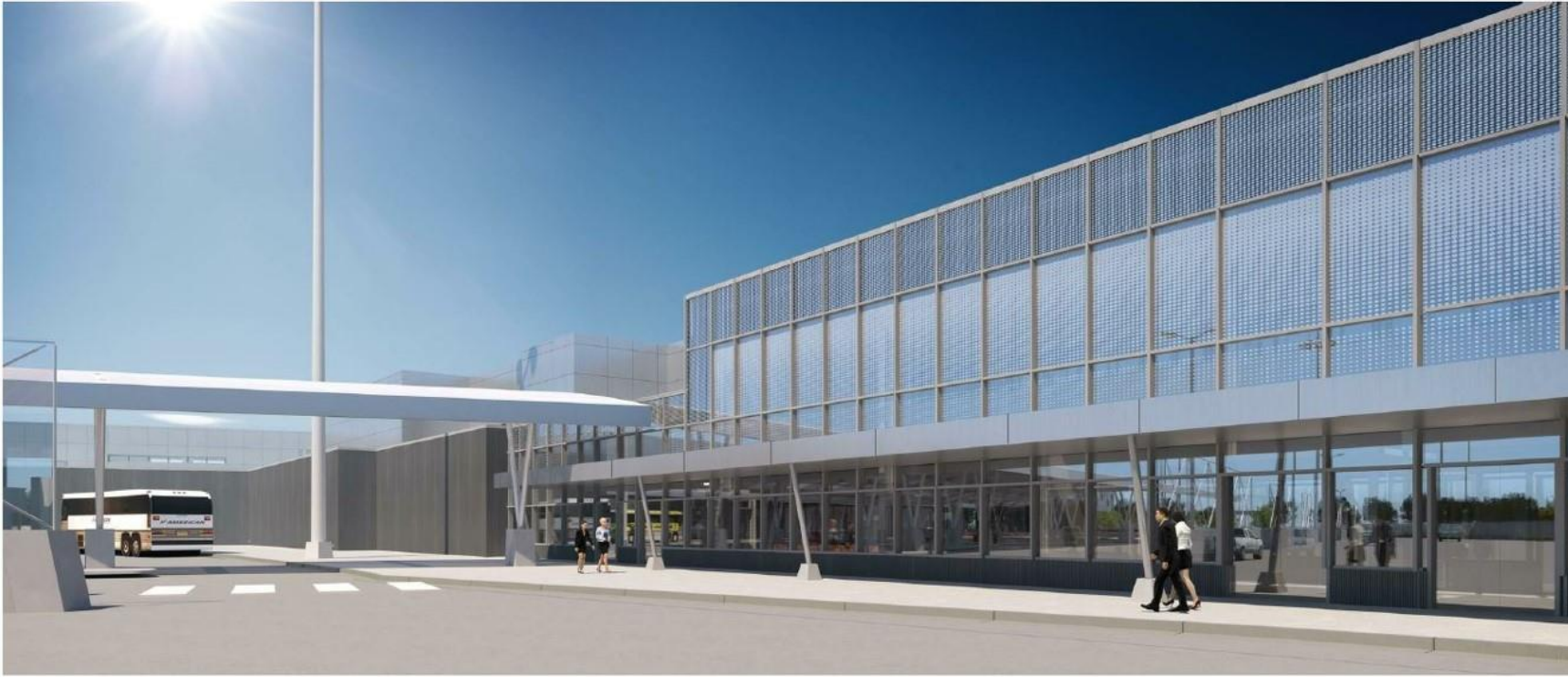
US POE administrative building from north
