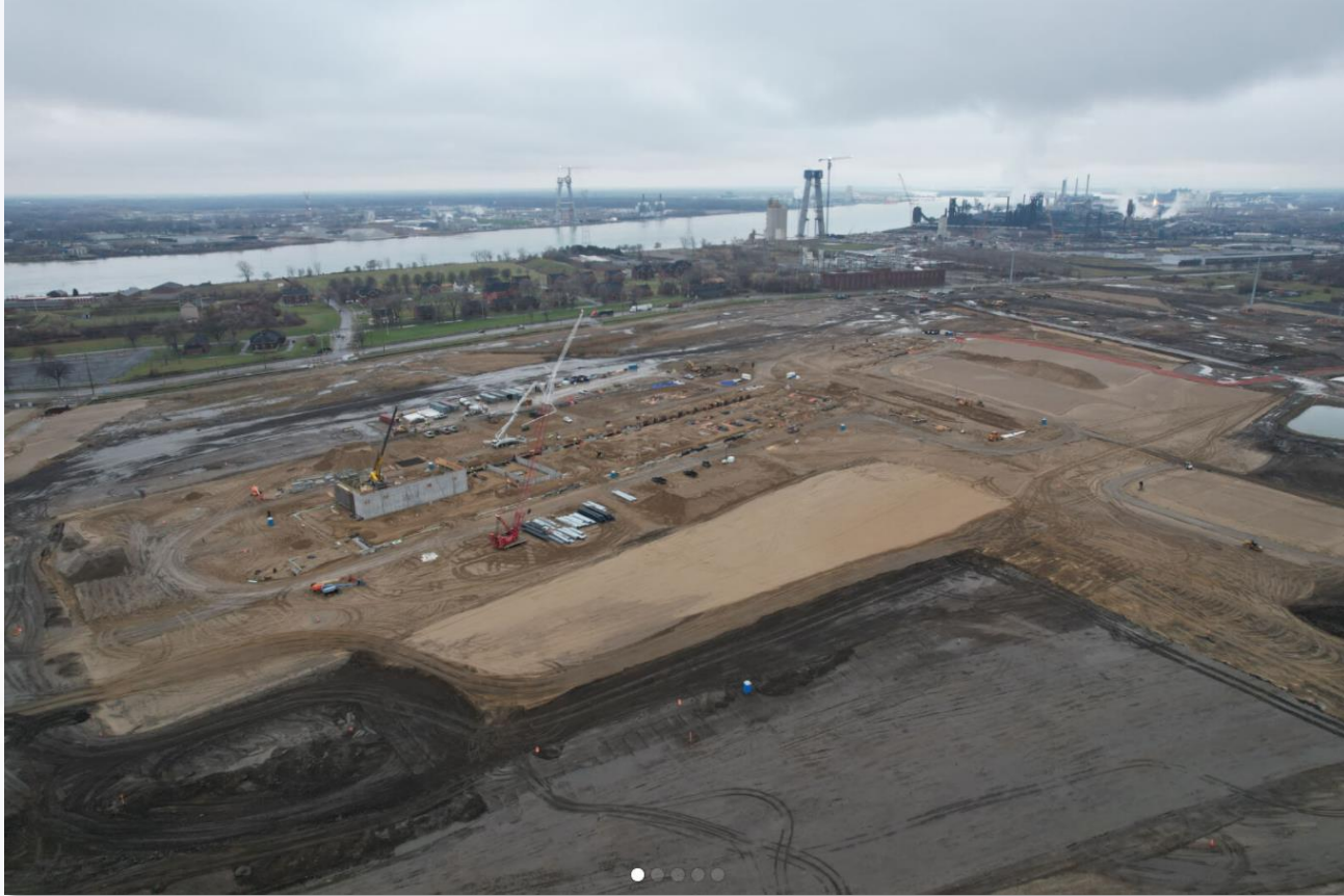
US POE construction site
