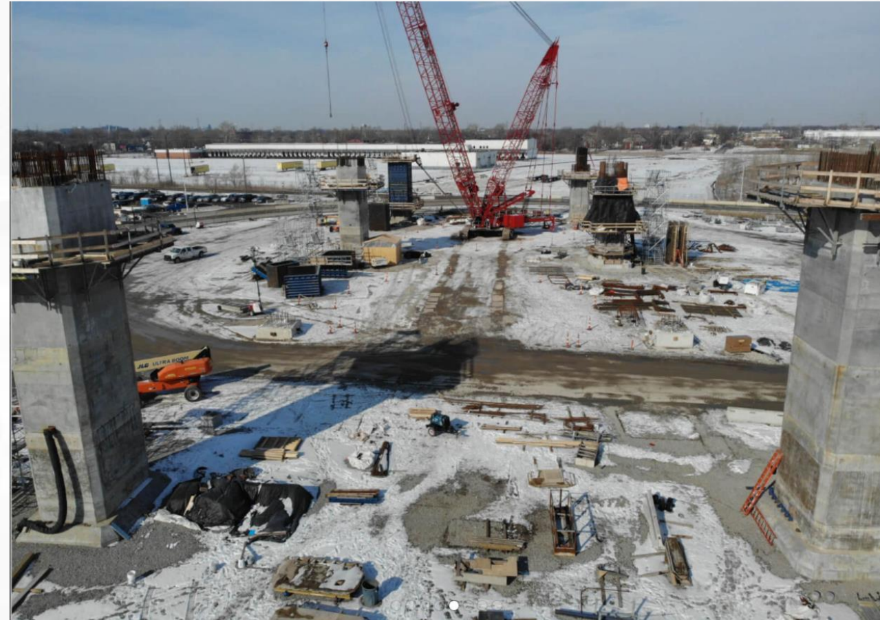
US bridge back span work
