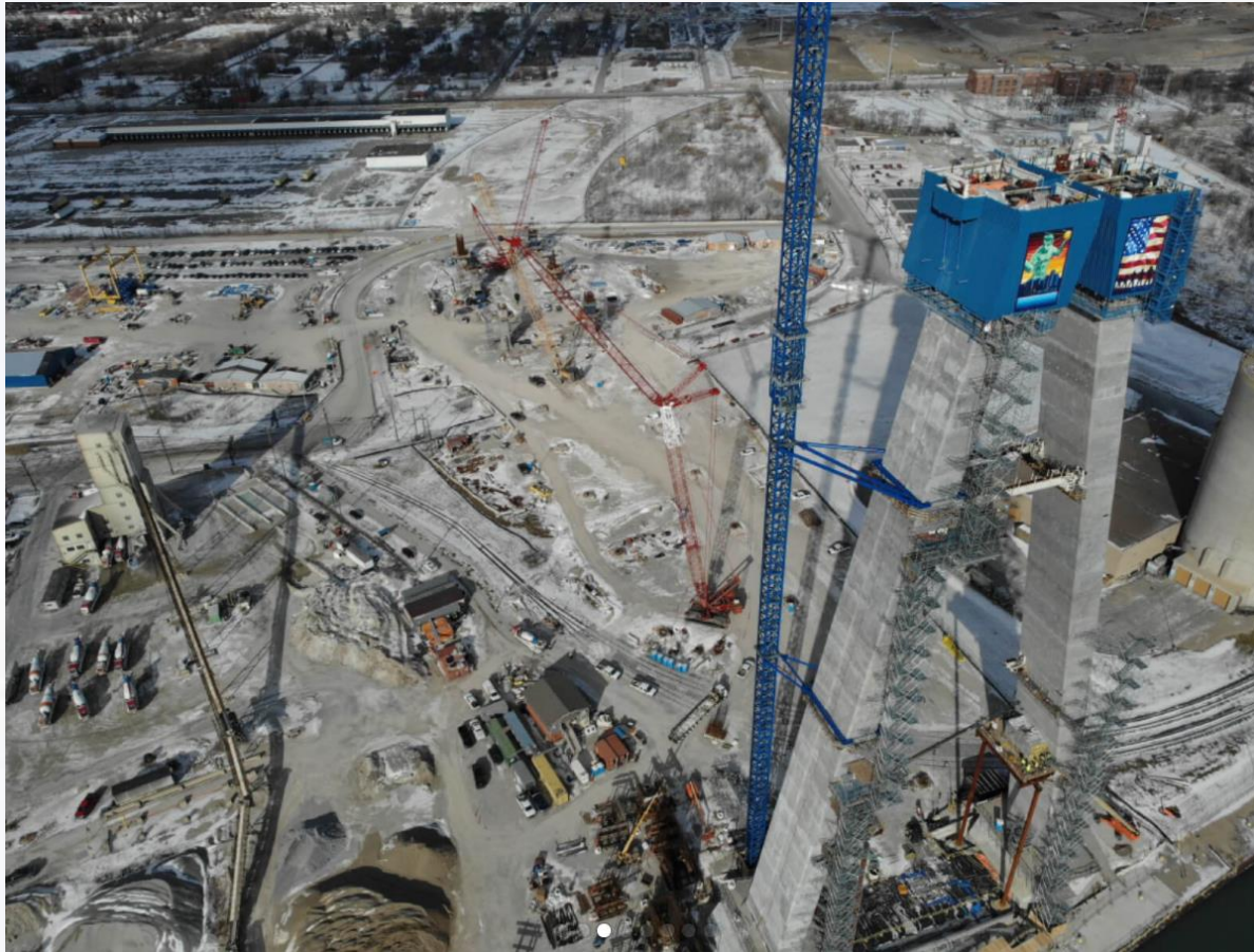
US bridge tower and back span work
