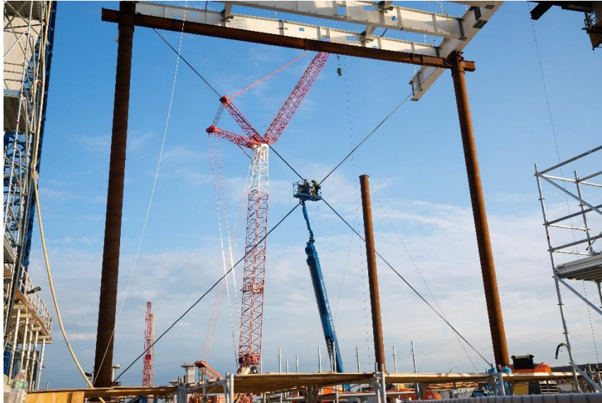
Workers are erecting the temporary falsework for the back span piers on the US bridge site.
