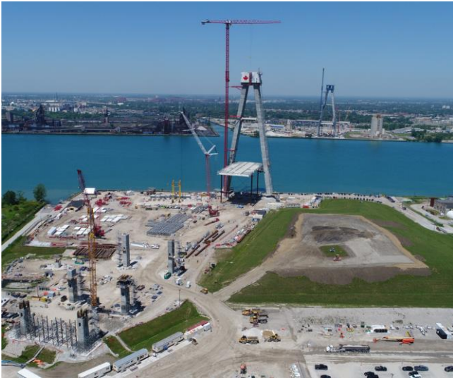
Canadian bridge deck and side span construction
