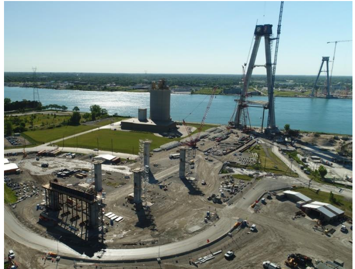
US bridge construction
