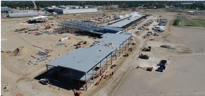
US Port of Entry facility construction
