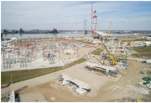
Canadian bridge site construction
