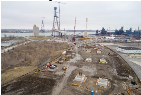
US bridge site construction
