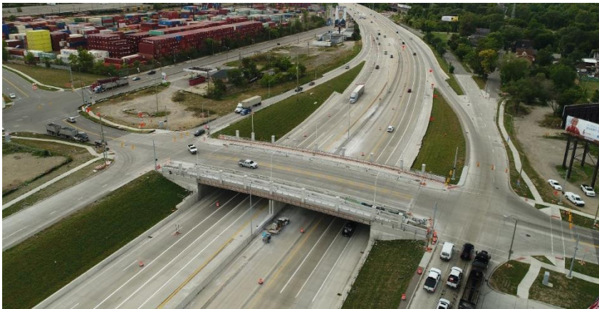
Springwells Street road bridge
