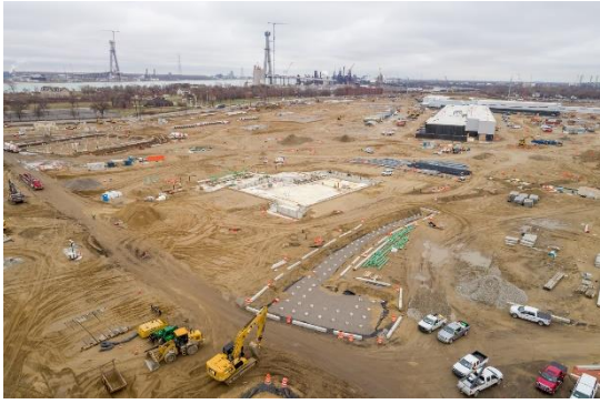
US Port of Entry construction
