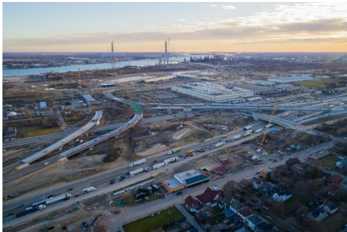
I-75 and US POE connector ramps construction progress
