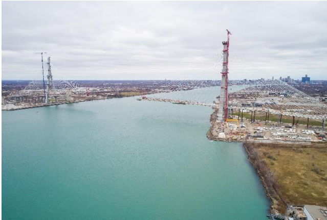
Bridge construction progress
