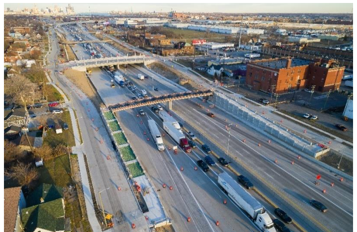
Solvay Street pedestrian bridge construction
