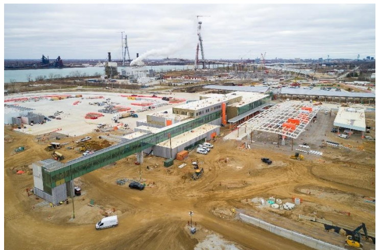
Canadian Port of Entry construction progress
