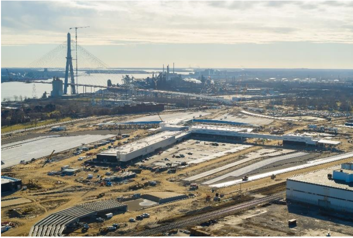
US Port of Entry construction progress
