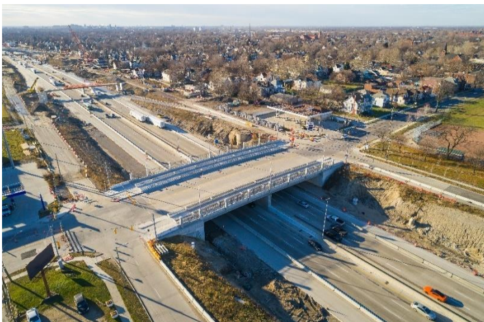
Clark Street road bridge
