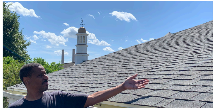
Forest Hudson shows off the gymnasium's new gabled roof at Delray Neighborhood House.
