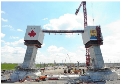
Canadian bridge tower work
