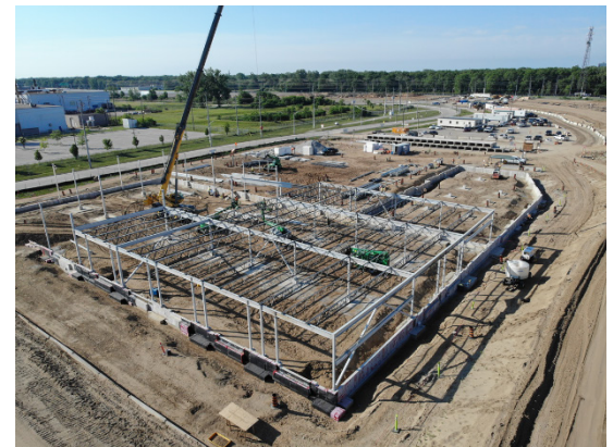
Building construction at the Canadian Port of Entry
