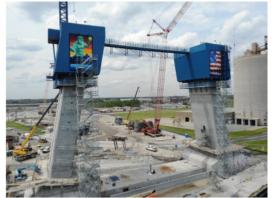
US bridge tower work
