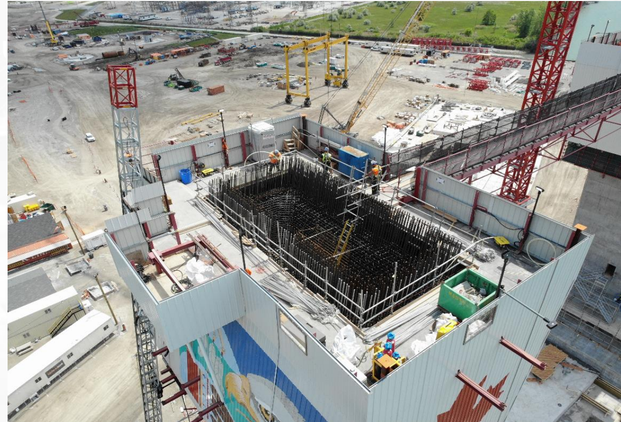
Canadian bridge tower work
