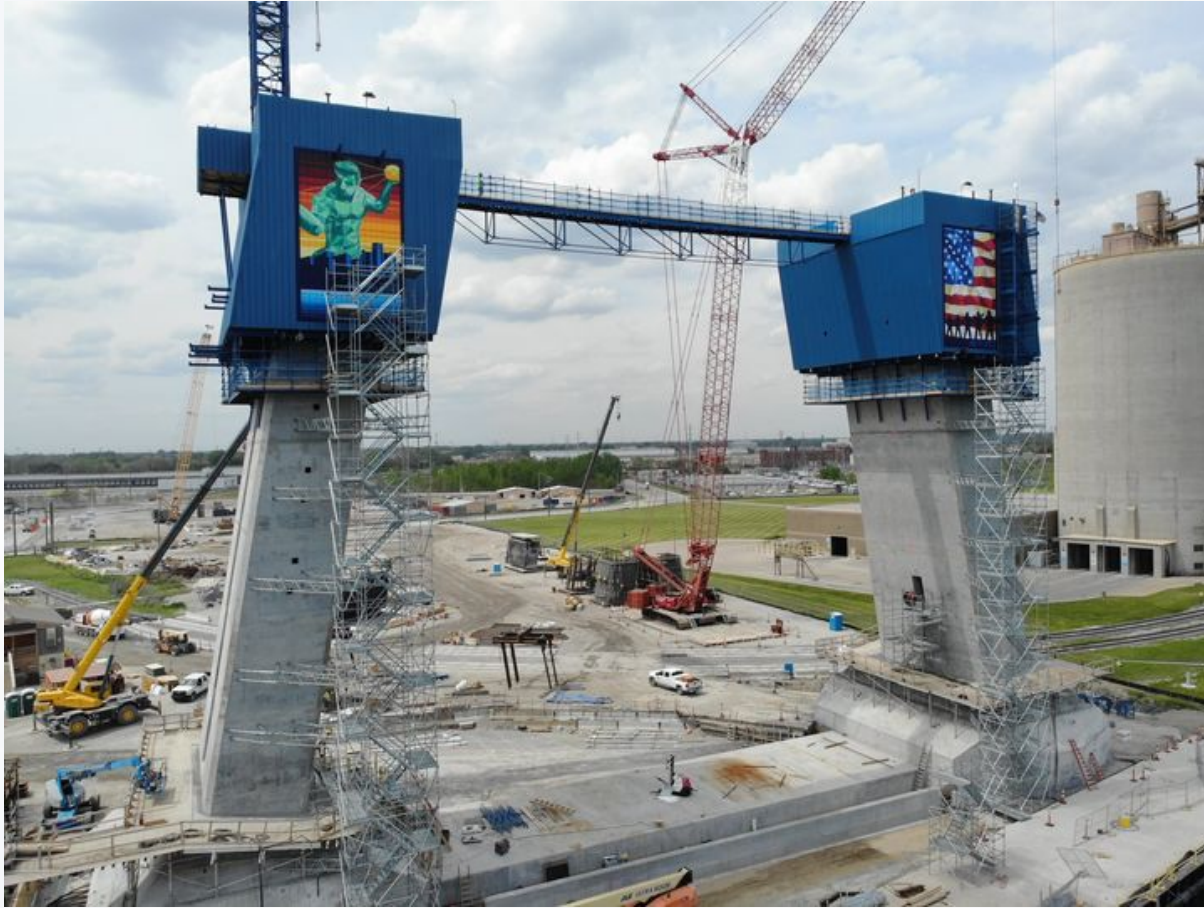
US bridge tower work
