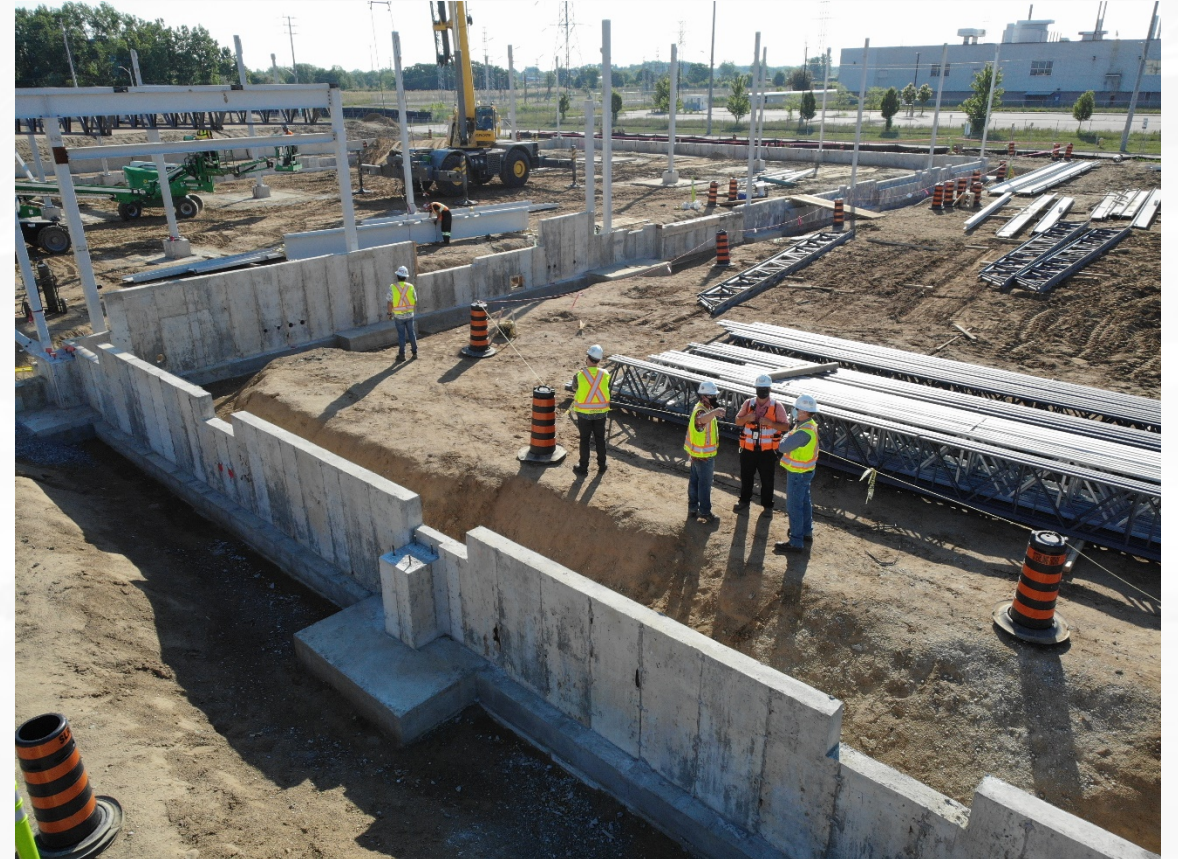
US POE building construction
