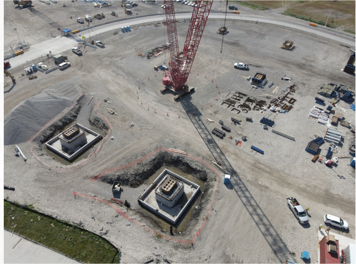
US bridge back span work
