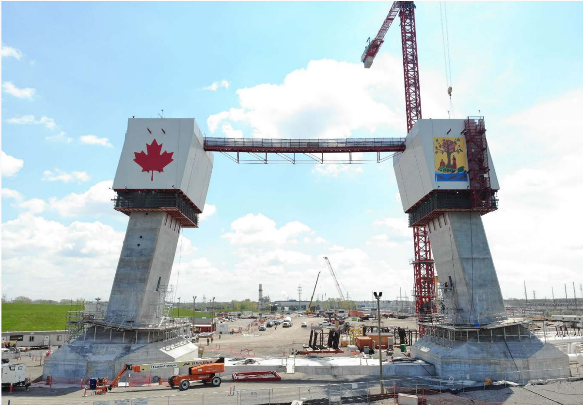
Canadian bridge tower work
