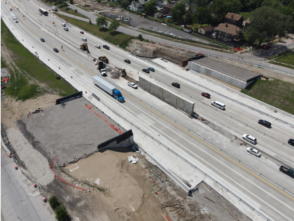
MI Interchange road bridge construction
