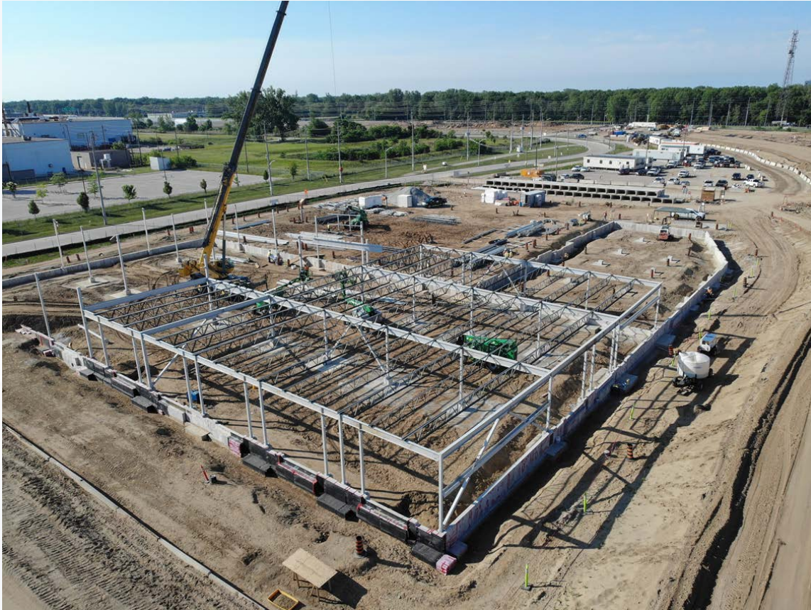
Canadian POE building construction
