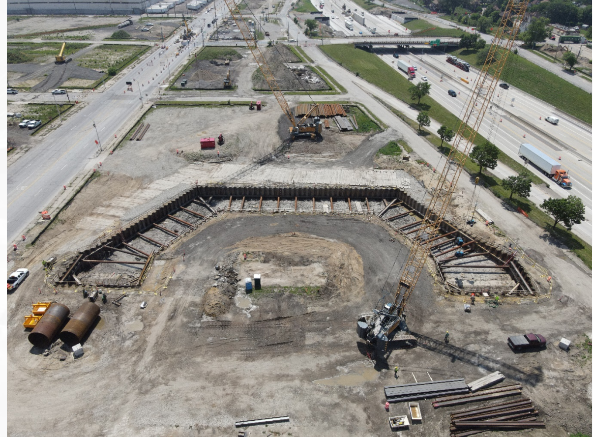
Cavalry siphon construction
