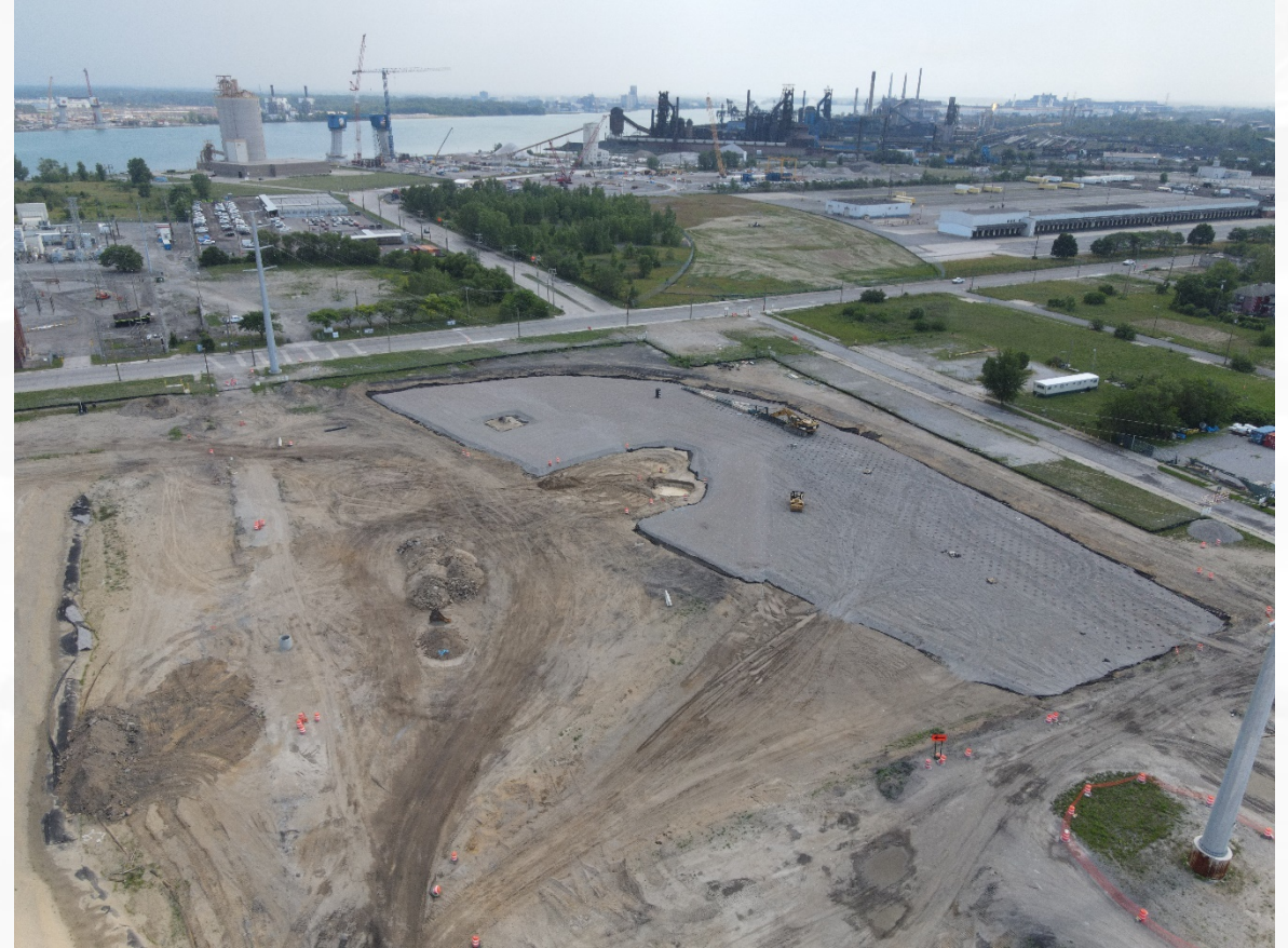
US POE wick drain installation
