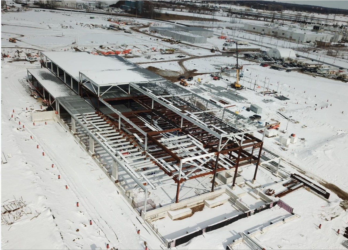
Canadian POE building construction
