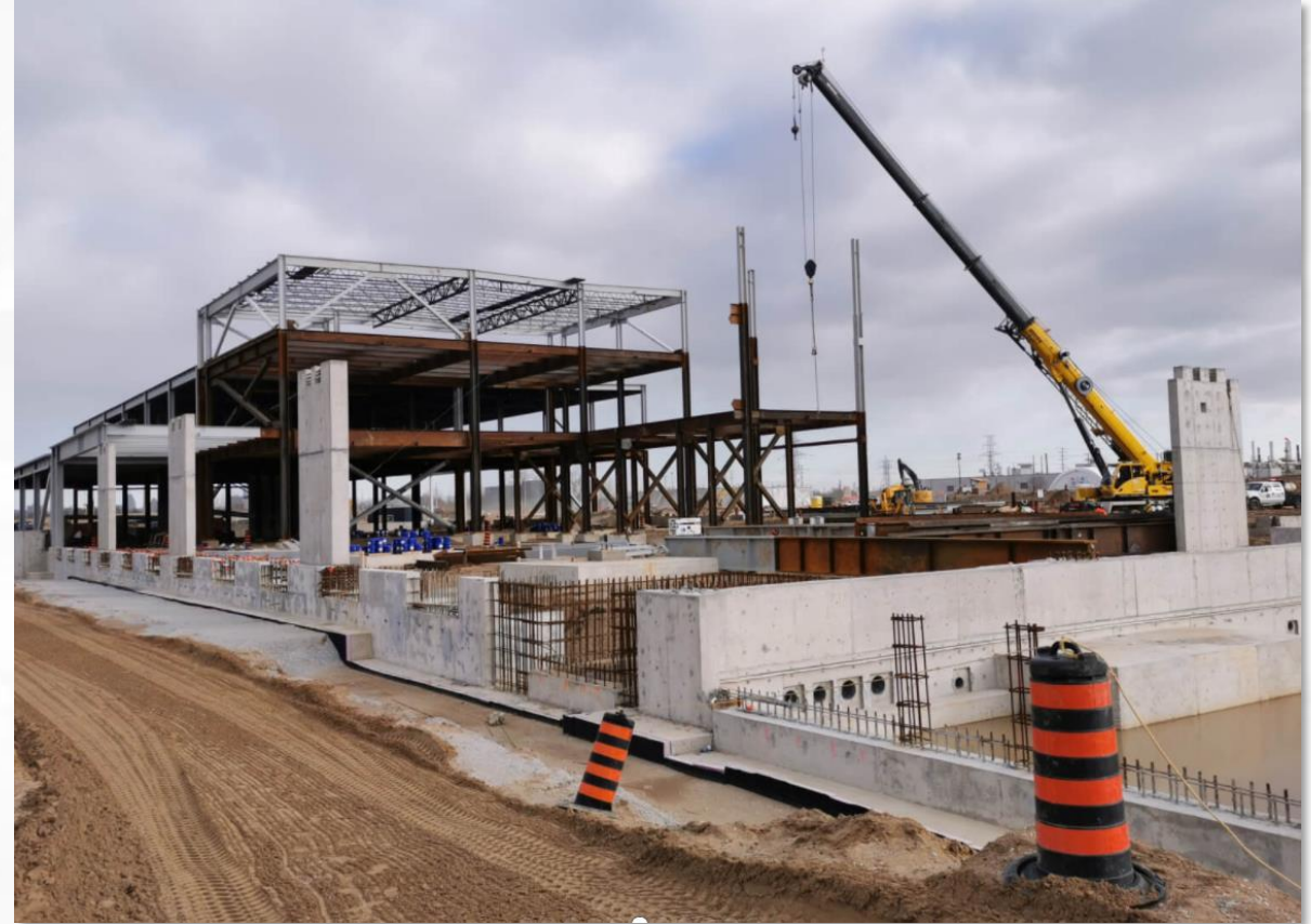
Canadian POE building construction
