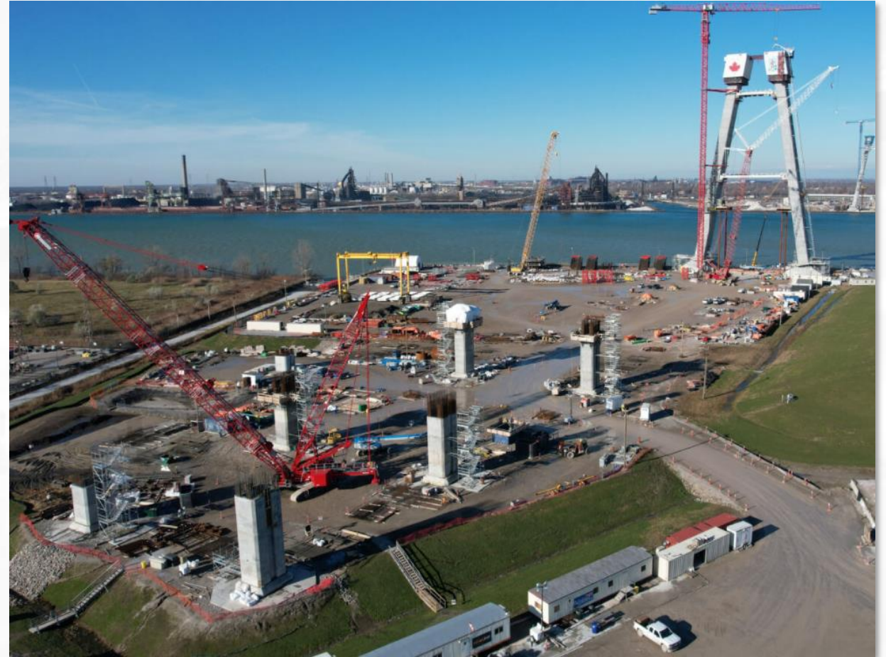
Canadian bridge back span tower work
