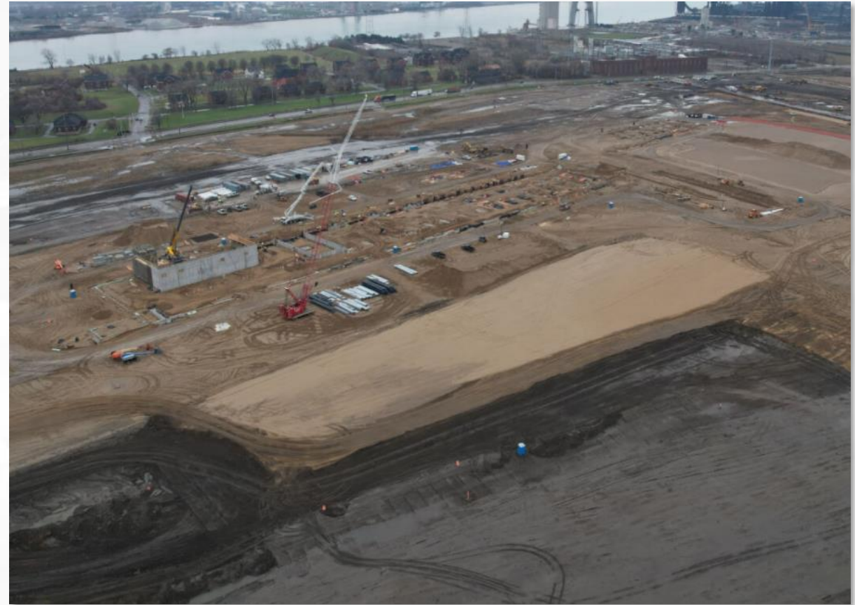
US POE building construction
