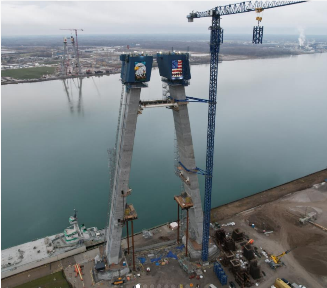
US bridge tower work
