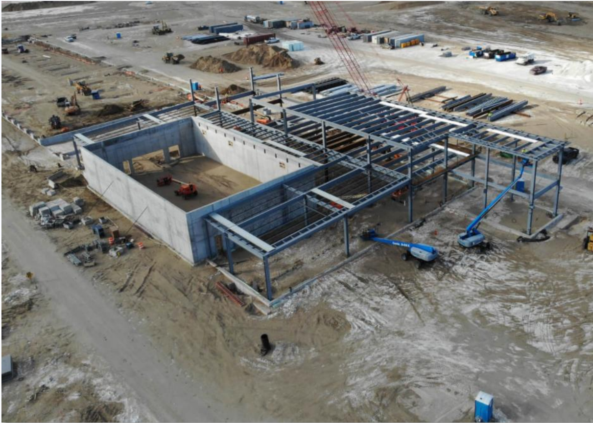
US POE building construction
