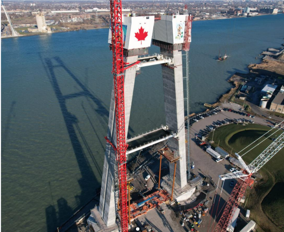
Canadian bridge tower work
