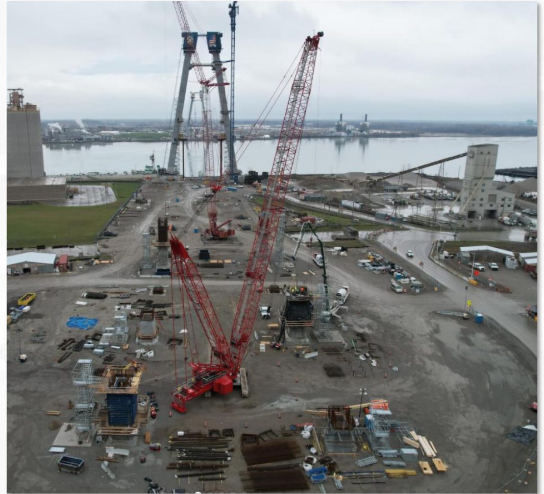
US bridge back span work
