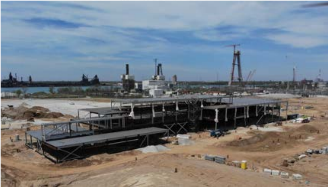
Above: Canadian Port of Entry, main building construction
