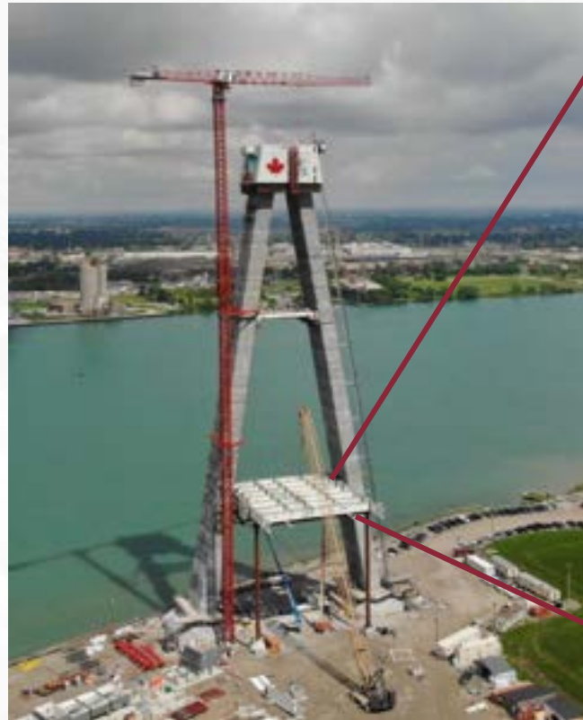
Left: Canadian bridge tower Right: bridge deck girder installation
