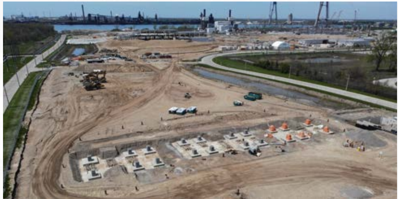
Above: Canadian Port of Entry, toll booth construction
