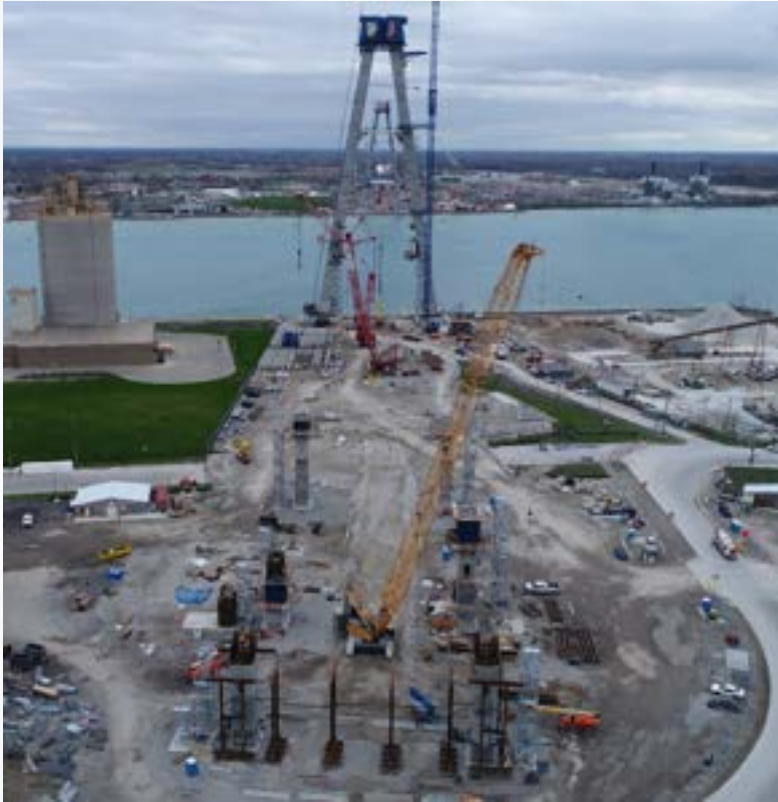
Above: US bridge site back span and bridge towers
