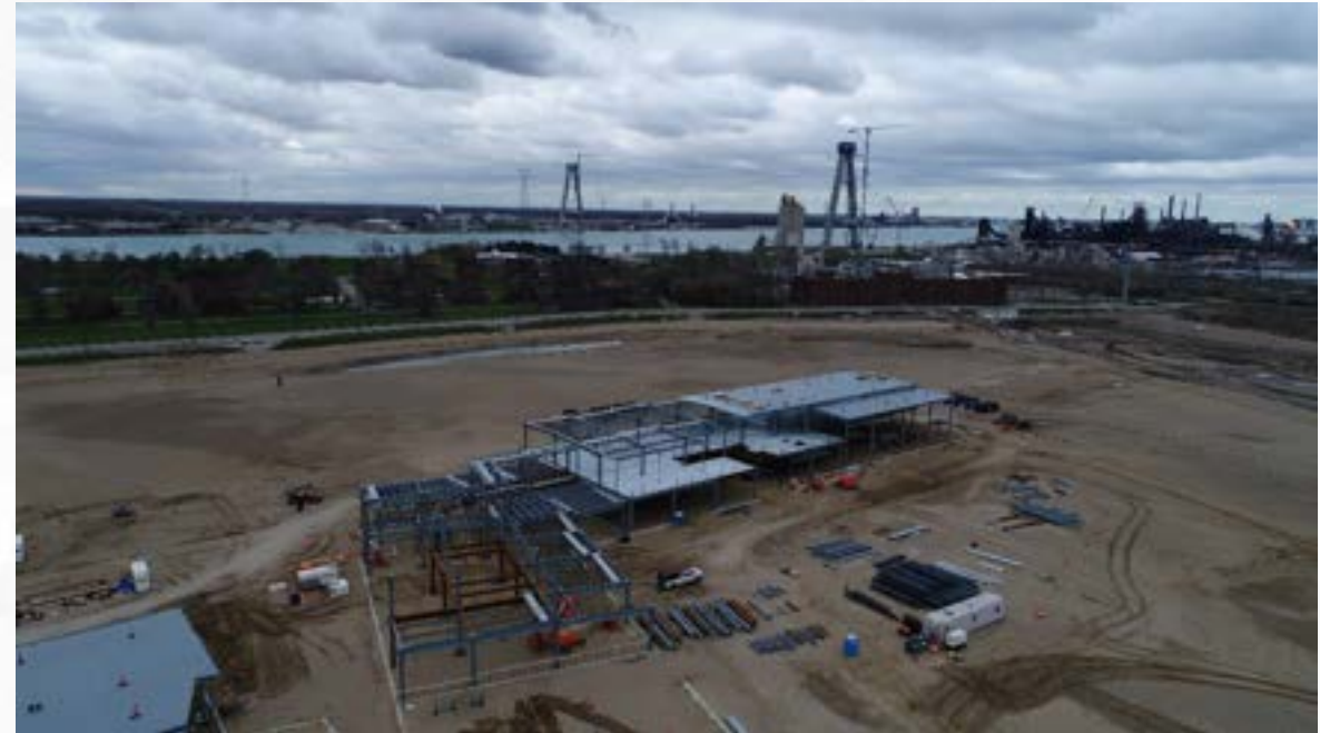
Above: US Port of Entry building construction
