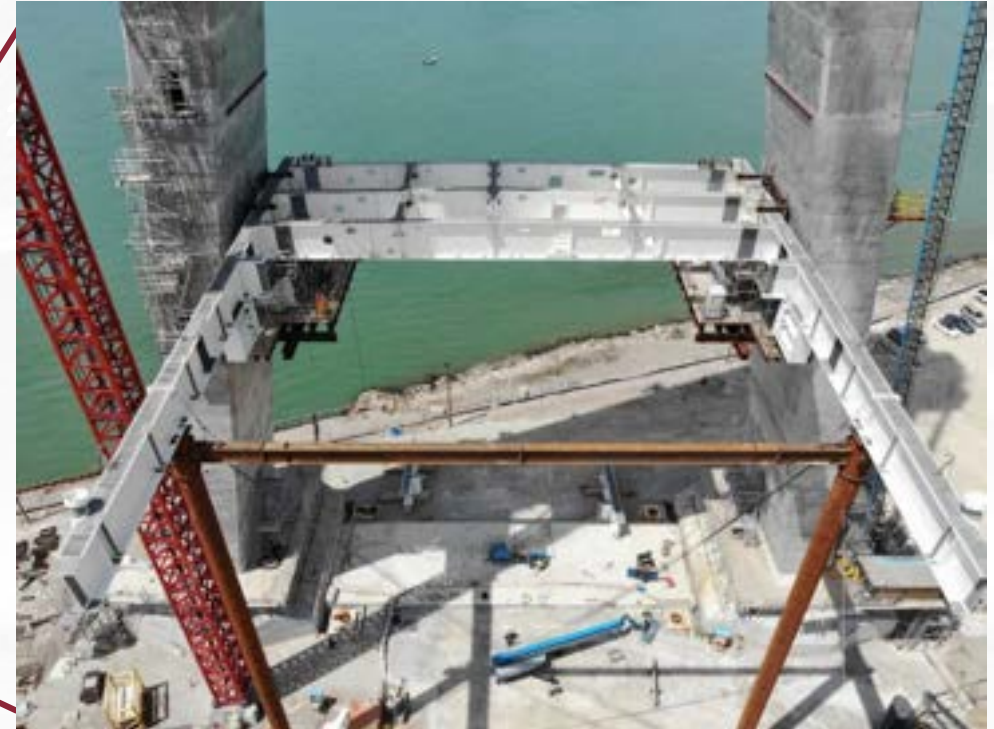
Left: Canadian bridge tower Right: bridge deck girder installation
