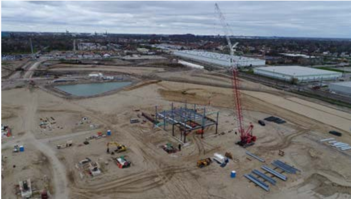
Above: US Port of Entry building construction
