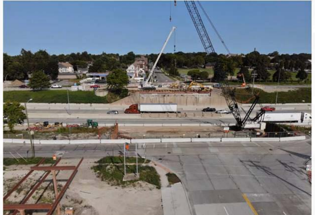
US Bridge Site
