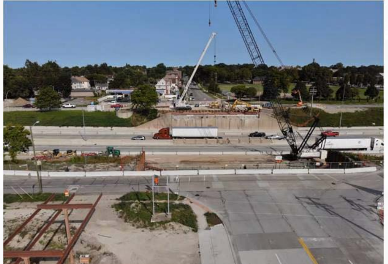
US Bridge Site
