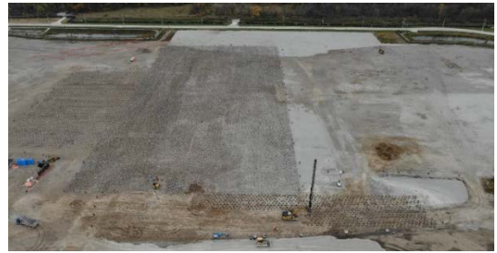
CDN POE wick drain installation
